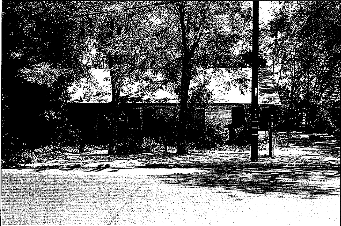
Left side facing north to 28th Street
